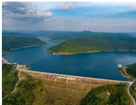
Photo: Cambodian Tatay Hydropower Station
