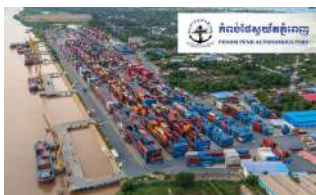
Photo: PPAP's Container Terminal LM17
