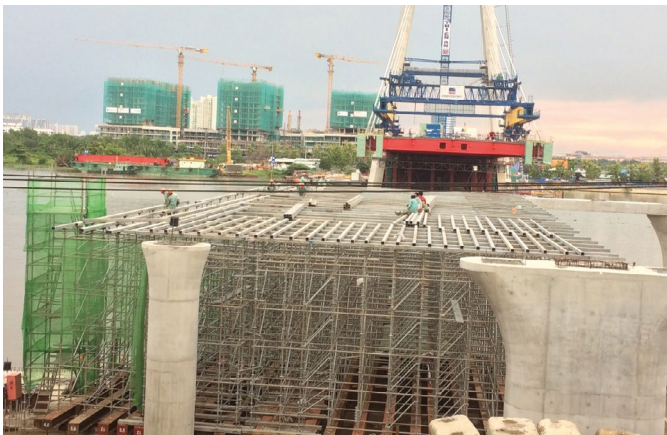
Falsework for a concrete bridge
