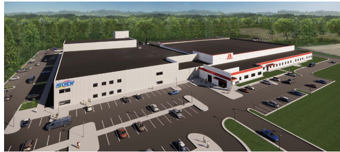
Morinaga America Foods Factory No.2 in NC, USA
