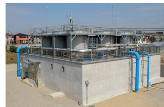
CHEMILES in operation Project of NAGAOKA
