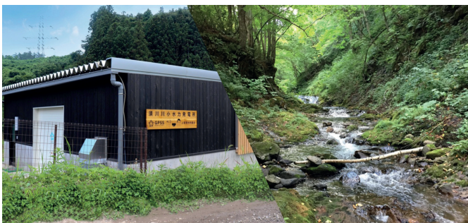
Sukawagawa small hydro power plant
