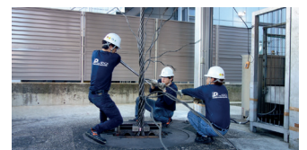
Hand splice for high-strength wire rope
