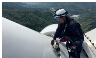
Installing blade on site
