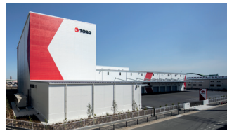
Automated warehouse in central Osaka, Japan
