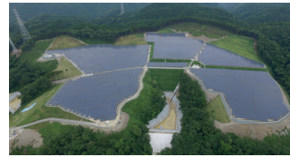
The Solar Panel Project Managed by JESCO
