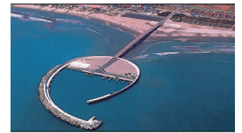
Wineglass-shaped Fishing Port designed as a solution to regional sediment transport problems
