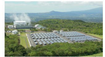
Costa Rica: solar power
