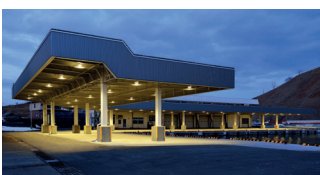
Fish landing and hygiene management facilities designed and built by AHEC
