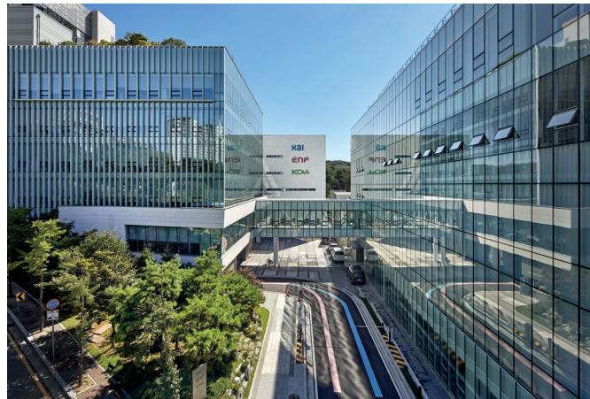
Headquarters building of ENF in Yong-in city
