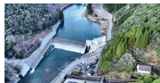
Hydroelectric power plant
