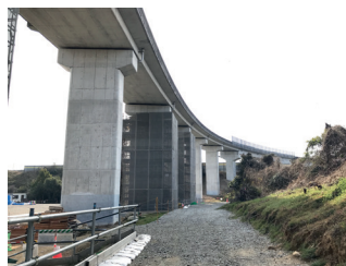
Highway bridge seismic reinforcement
