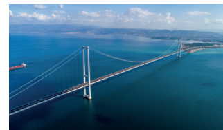
Osman Gazi Bridge, Turkey
