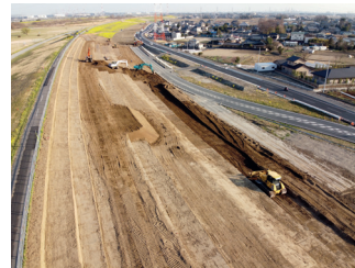
Levee protection works
