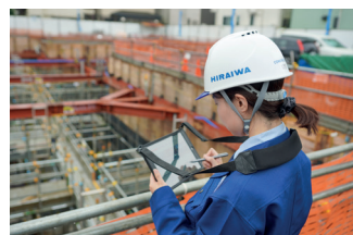
Women play an active role at construction site
