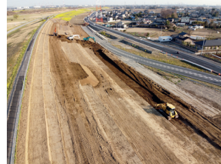
Levee protection works
