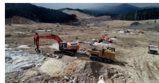
Large land reclamation and formation
