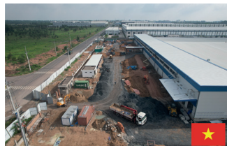
Factory construction in Vietnam
