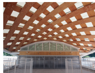
JR Onagawa St. (LVL), Miyagi, Japan
