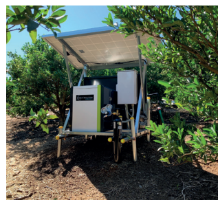
Off-grid NB generation from solar panels
