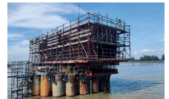
Bridge construction project in Bangladesh
