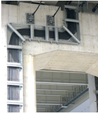
Electrical wire duct installation on a highway
