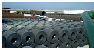
Pipeline project in Qatar
