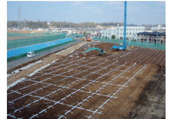
PVD ground improvement
