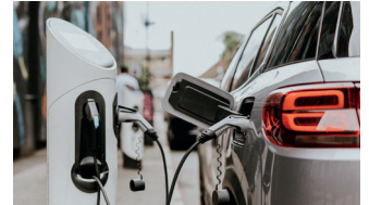
EV charging station
