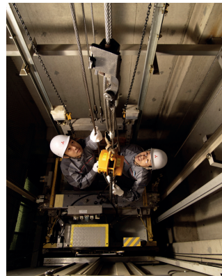
Inspection in elevator shaft
