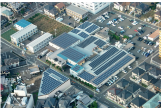
Rooftop solar panels at TSUBAME TOWEL Co., Ltd.
