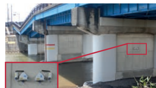
Remote Monitoring Device on Bridge Pier
