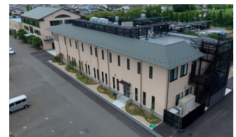
New Testing Building
