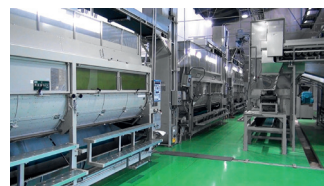
Tea processing plant
