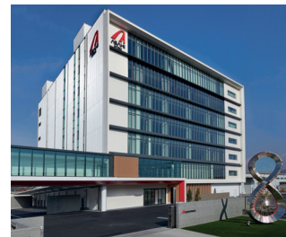
Asahi Intecc Co., Ltd.'s global headquarters and R&D center
